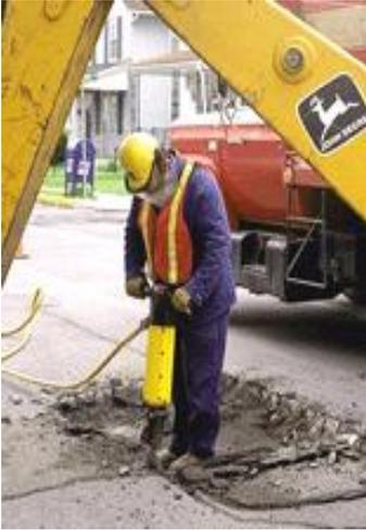
Pneumatics typically comes in three sizes 20 lb., 60 lb., and 90 lb. weight class. Pneumatics hit harder than the electric version and as a result breaks thicker material in less time. All of the pneumatics mentioned requires a tow-behind air compressor with 100-185 cfm.
