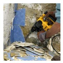
These are small hand-held breakers that can be fitted with many different types of bits such as points or chisel for breaking concrete, wide blade chisels for tile removal, and drill or coring bits ranging in diameter from ½"-6" in diameter.
